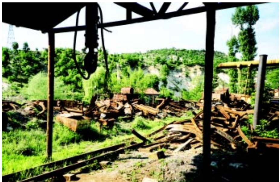
Abandoned surface facilities at the Pirin Mine
