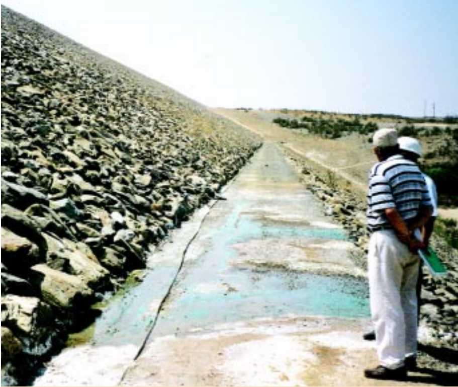
The tailings is placed sub-aqueously behind a rockfill embankment
