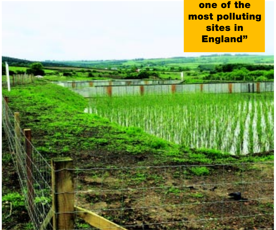
The Edmondsley wetland uses reeds to filter metals which precipitate from the water
